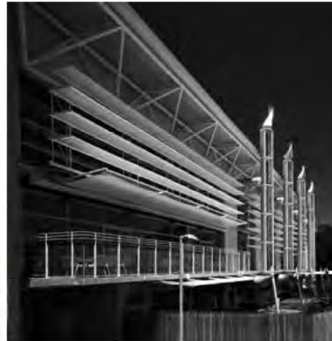
top: diagrammatic representation of the Concord Library Centre's naturally driven ventilation and cooling system; right: view of northern facade showing the thermal chimneys which drive the building's ventilation system
